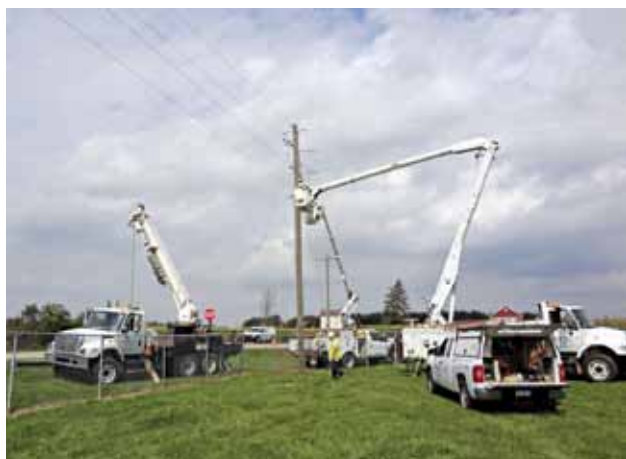
Crews work together to replace a broken pole.
