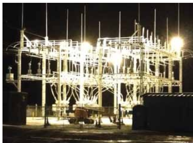
Construction to upgrade the Portland substation sometimes took place at night.
